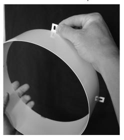
**Step 2:** Remove the adhesive from the foam tape. Adhere the foam around the inside of each 10" collar - cut off any access foam tape.
