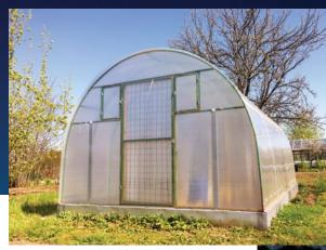
Because of its clarity, plants grown under glass glazing are more prone to leaf burn and other light-induced stressors than plants grown under polycarbonate or plastic films. Glass greenhouse owners and managers have gotten around this by using shading compounds (see below).
