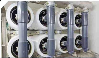
**Osmosis** refers to the diffusion, or flow, of liquid moving through a selectively permeable filtration membrane. In growing, the process of **reverse osmosis** is typically performed through the use of a specialised filtration system. This process is used to clean water so it's better suited for effective irrigation. In fact, reverse osmosis can remove all the dissolved solids from water, leaving pure H<sub>2</sub>0, which allows a grower to more accurately control nutrient dosage and uptake.
