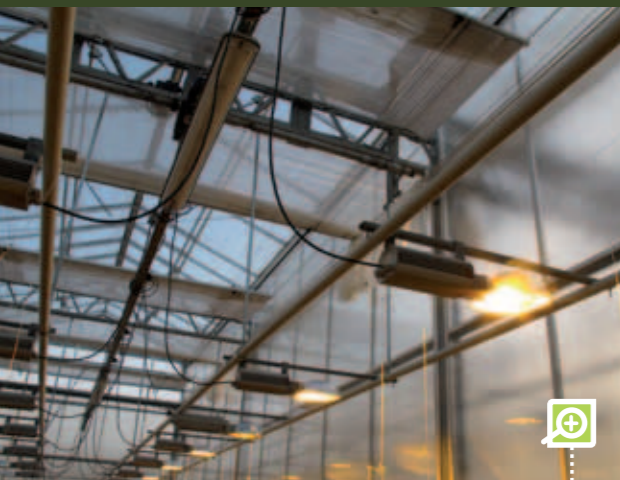
Figure 10: High pressure sodium lamps in a greenhouse
